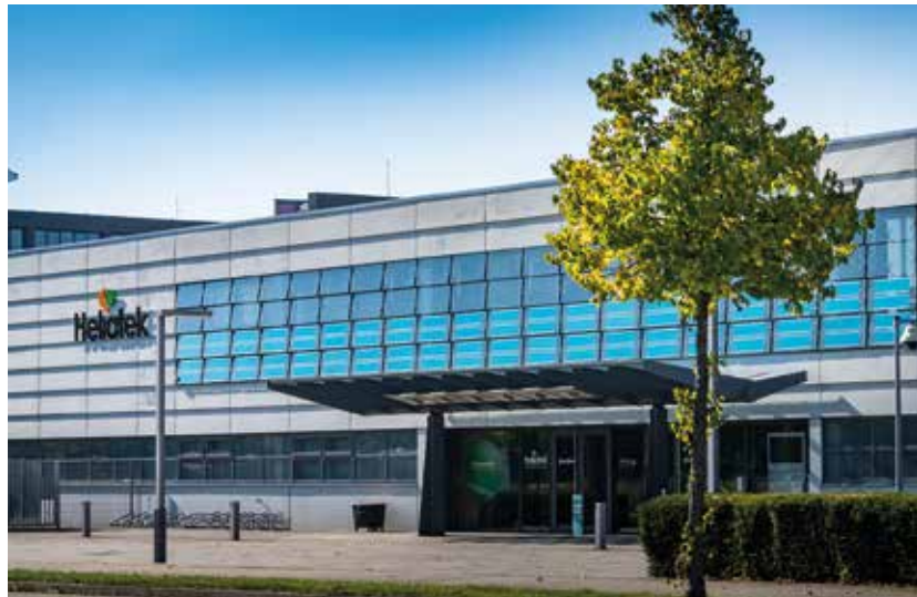
Fig. 1: Solar Glass Façade in Dresden North-East orientation to test low light behaviour 1 kWp
