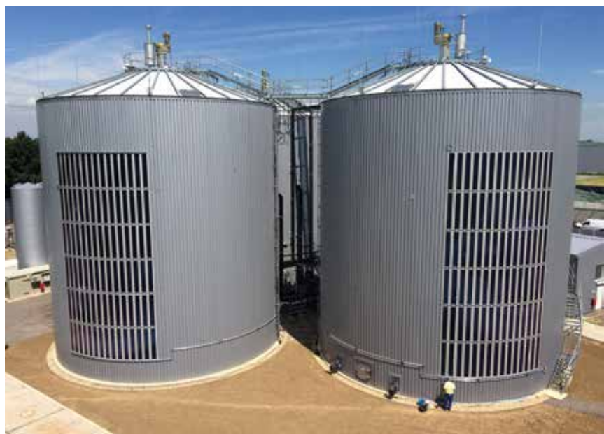
Fig. 5: Innogy plant with organic solar films by Heliatek
